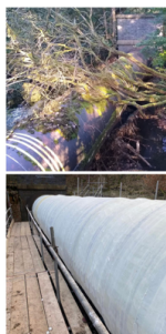
2) Tightly wrap the bandage around the pipe
