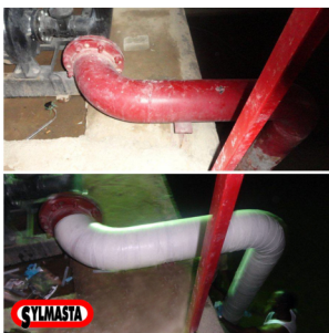
1) Use water to activate the resin
