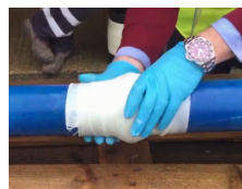
3) Smooth and tighten the bandage onto the pipe
