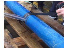
2) Stretch tape to exert maximum pressure
