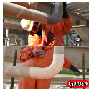
4) The repair will set rock-hard once complete
