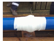
4) The repair will set rock-hard once complete
