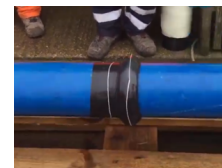
4) The tape fuses, sealing the leak
