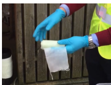
1) Use water to activate the resin
