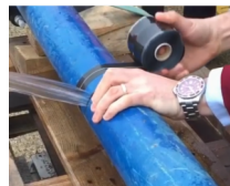
1) Anchor the tape next to the leak area
