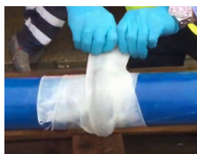
2) Tightly wrap the bandage around the pipe
